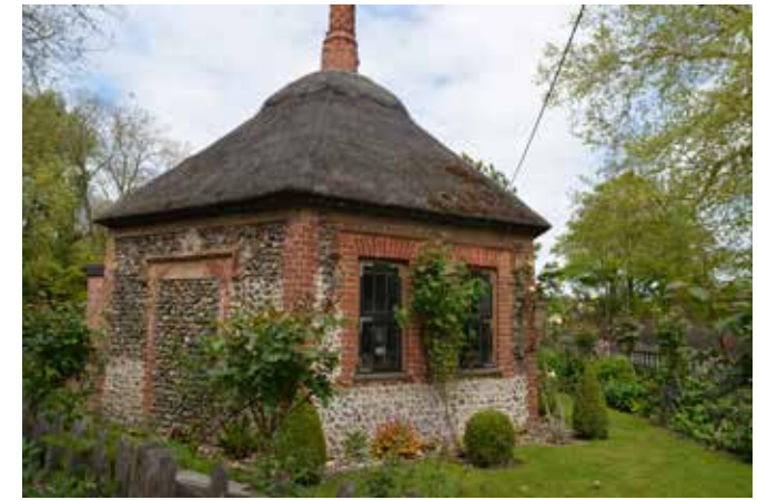
Figure 45: St Johns Well Cottage, a Grade II listed building.
