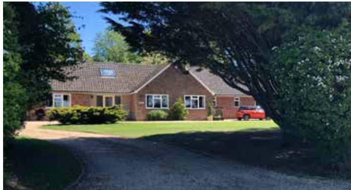
Figure 20: 1.5 storey bungalow on The Park.
