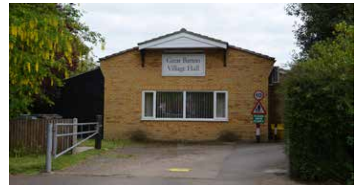
Figure 16: Great Barton Village Hall on Elms Close.
