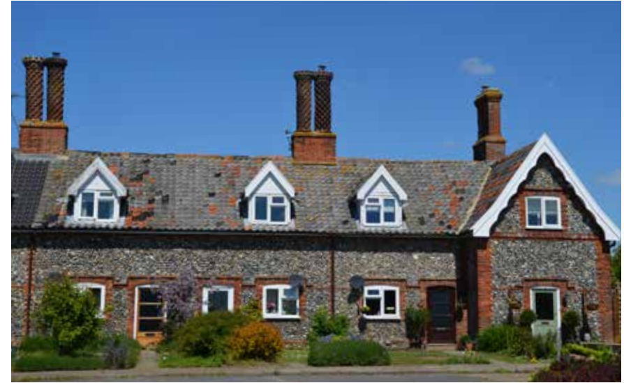
Figure 93: Historic building with cross gabled roof and dormers.
