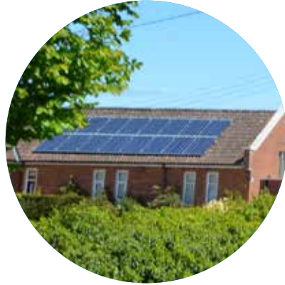
SOLAR PANELS, ALTHOUGH THEY SHOULD BE LESS INTRUSIVE THAN HERE
