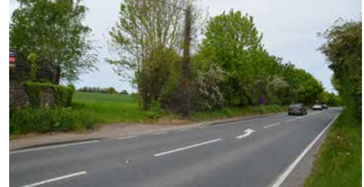
Figure 28: The Street (A143) - an example of a primary road.
