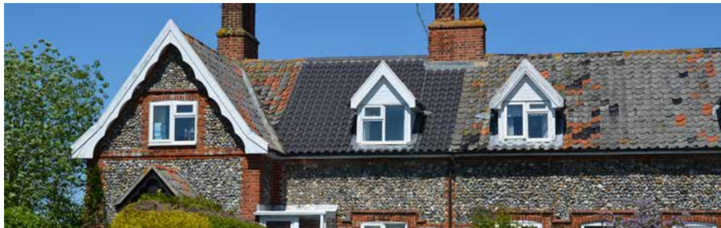
Figure 40: Shinham Bridge, historic terrace of houses.
