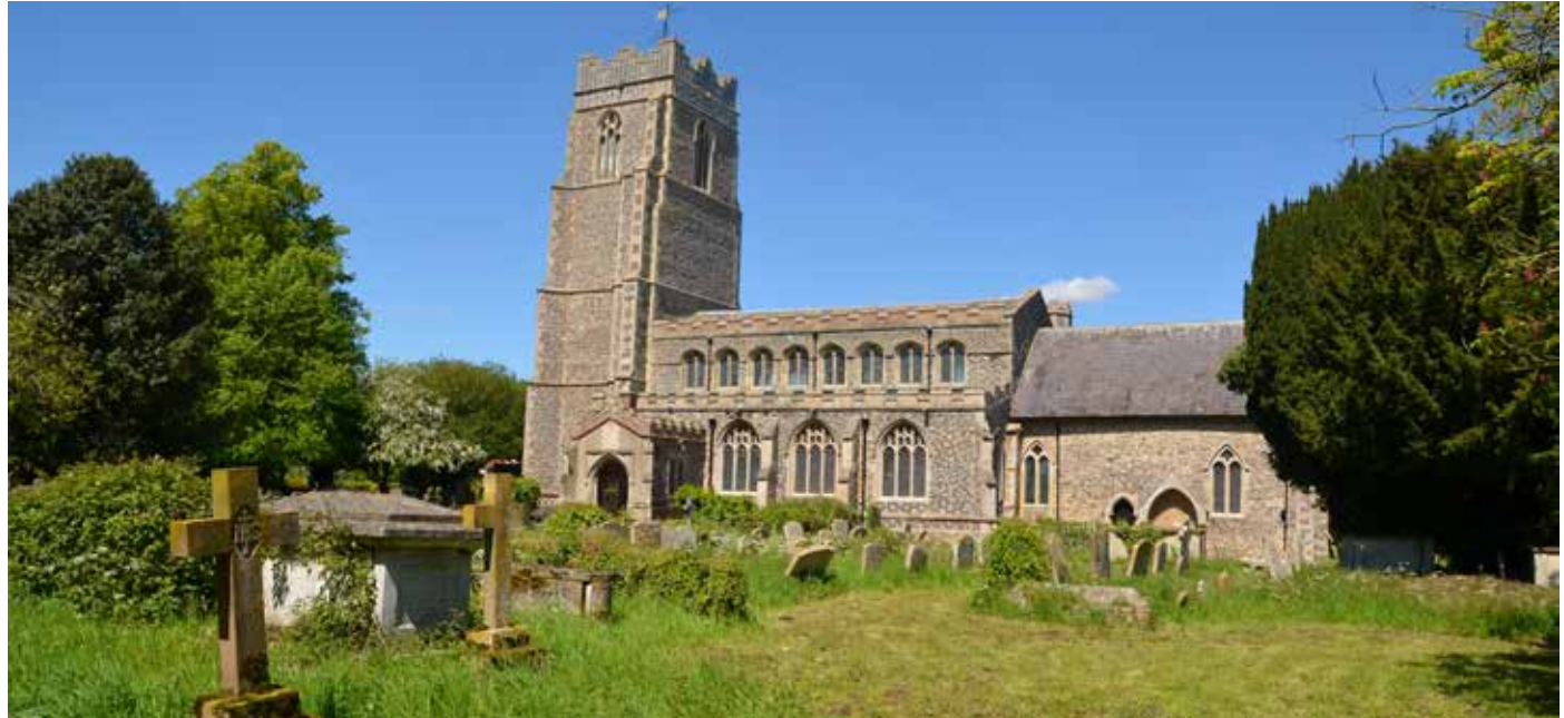
Figure 41: Holy Innocents Church Great Barton, a Grade I listed building.
