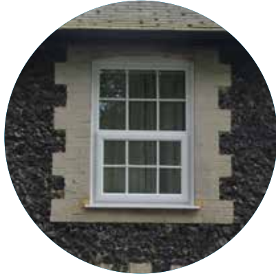
MASONRY DETAIL AROUND WINDOW
