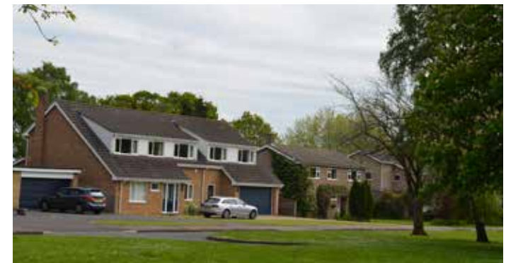
Figure 18: Two-storey building on Bunbury Avenue.
