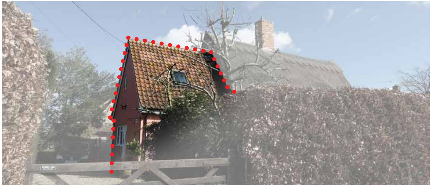
Figure 93: An example of positive design for contemporary side extension, habitable space and garage amenity.
