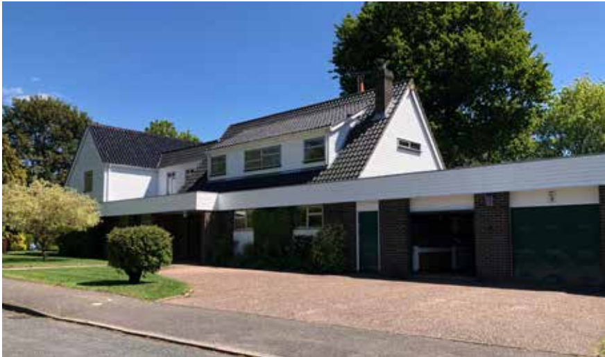
Figure 5: Modern architecture on Diomed Drive.
