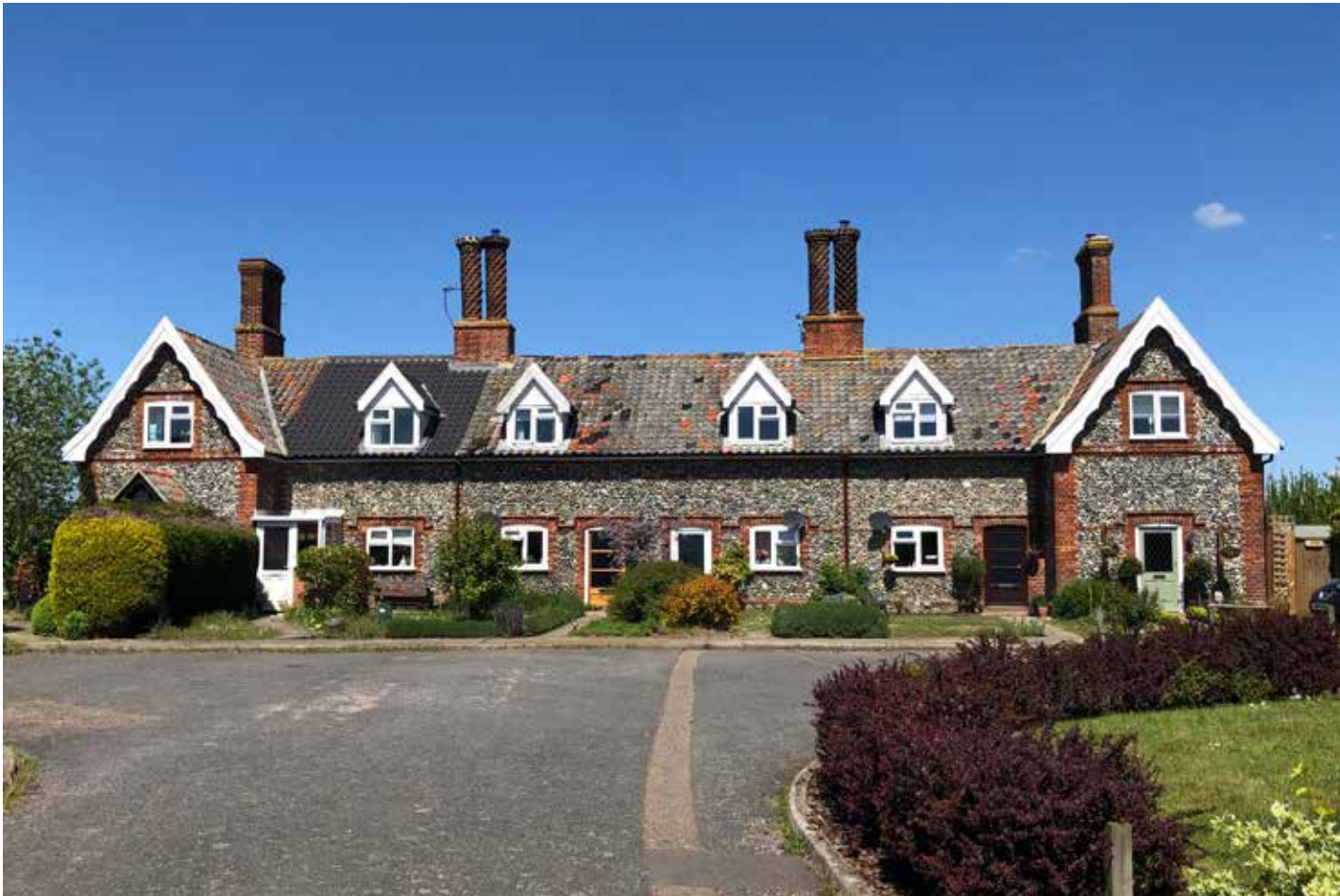
Figure 7: Cottages with distinctive chimneys on Shinham Bridge.
