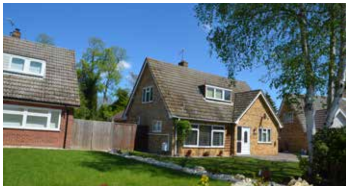
Figure 2: Detached buildings along Conyers Way.
