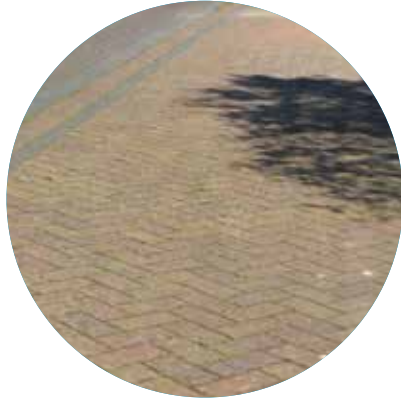
HERRINGBONE BRICK PAVING
