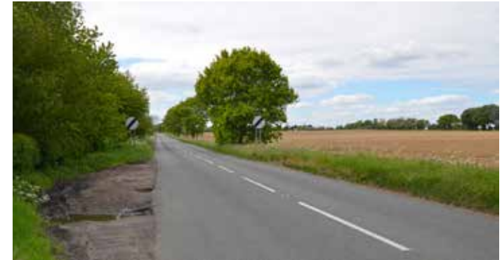
Figure 26: Mill Road - an example of a secondary road.
