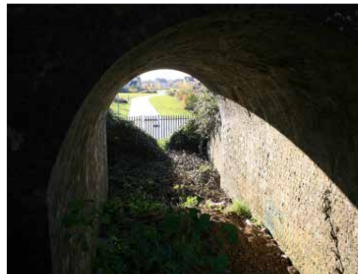
Image 15: Closed off Underpass Access under Railway
